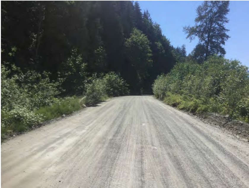
Approach from Right Bank when facing downstream
