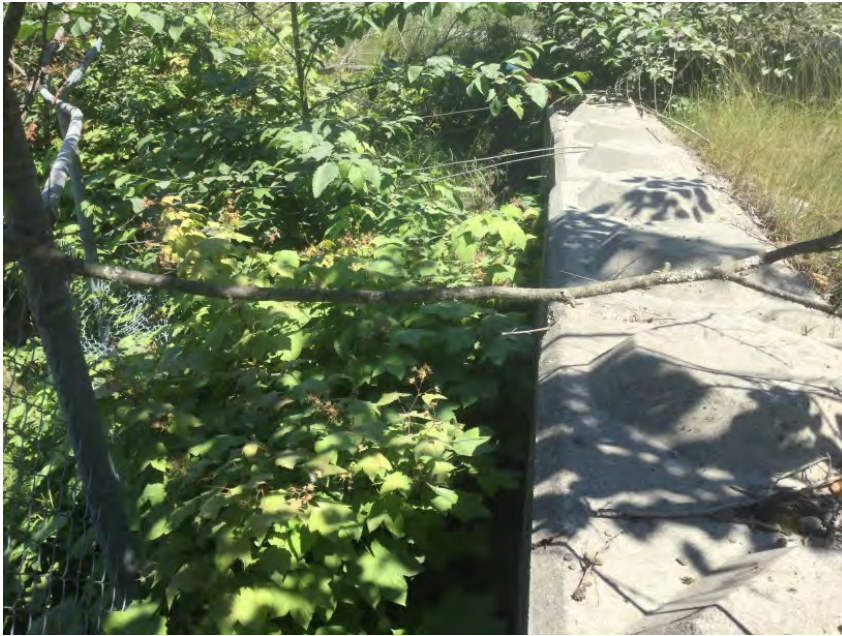
Downstream wall retaining fill
